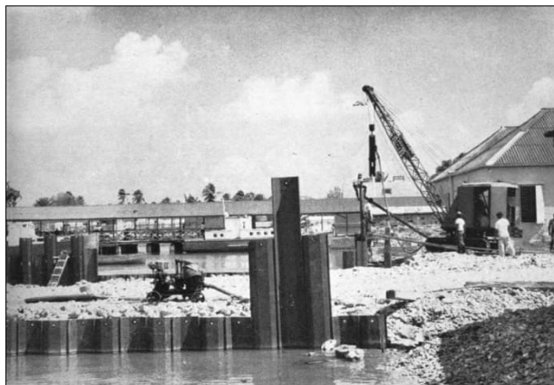
Construction work on extension of St. John's wharf 1960's
